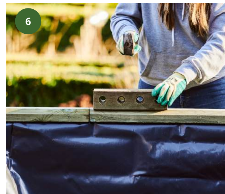
Knock on your capping layer - use a spare BlocX to protect the wood when hammering. JOB DONE!
