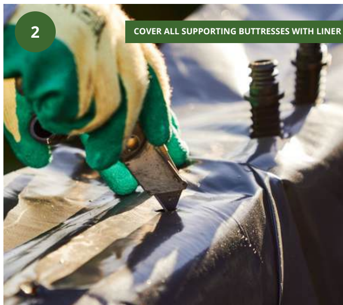
Get your liner into position - make small incisions for the final layer dowels to push through the liner.
