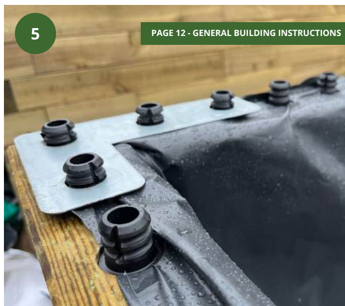
Install your angle corner plates - use your dowel protector to hammer these plates firmly into place.
